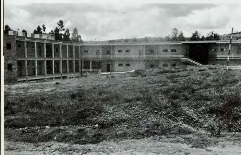
The back view of the main classroom building. Because of the ideal climate, the corridors are all opened.
