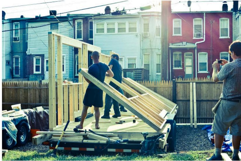
Image: Raising the interior wall of the “Matchbox” tiny home, built on a trailer bed
